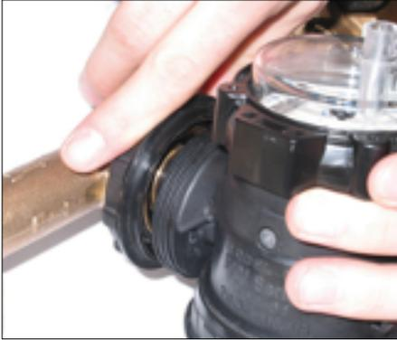
3. Position FAM Measuring Unit to Flow Tube; be sure the Measuring Unit is seated properly when mated with Flow Tube and that it is vertically level.
